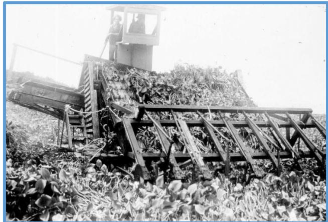
Top: A mechanical harvester removes *Ludwigia* spp. (water primrose) from a Florida lake, 2014. Above: A mechanical "hyacinth rake" removes *Eichhornia crassipes* (water hyacinth) from a Florida lake, circa 1930s.
